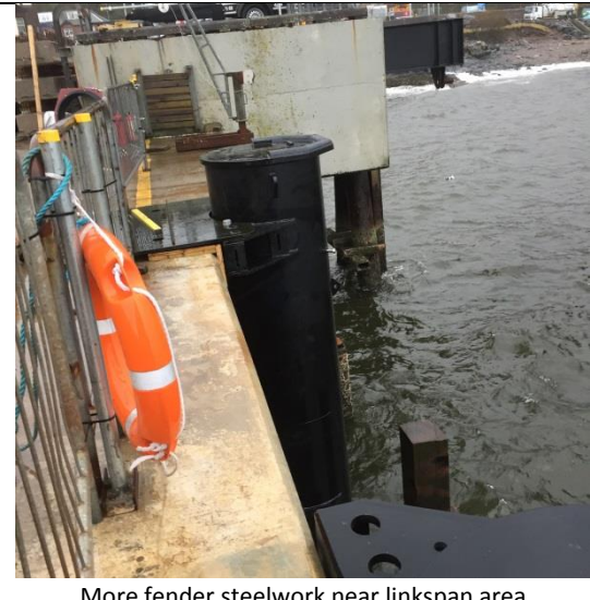
More fender steelwork near linkspan area
