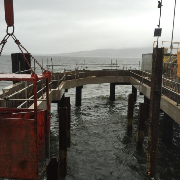
New roundhead ring beam units installed
