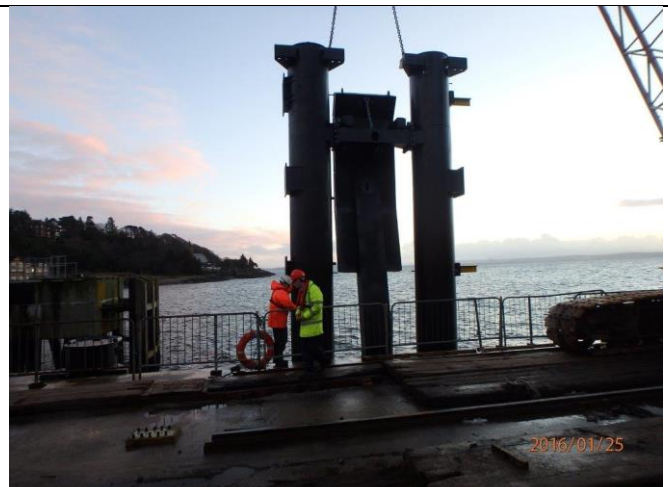
Fender unit being installed at Wemyss Bay
