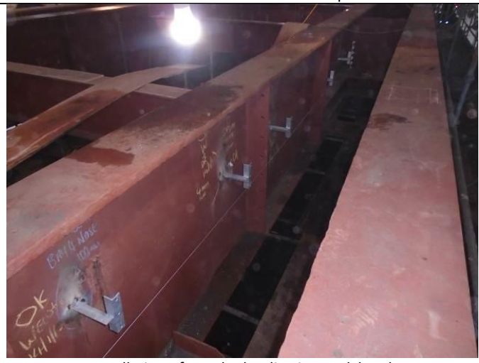
Installation of new hydraulic pipework brackets
