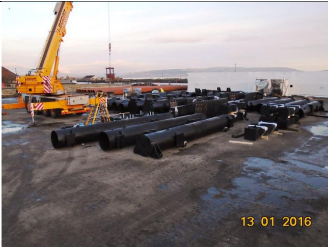
First fender delivery at Inchgreen
