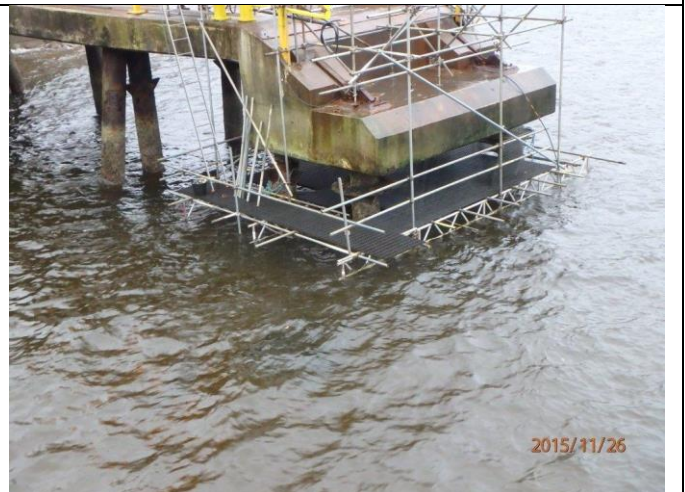
View of Bankseat Repair Area
