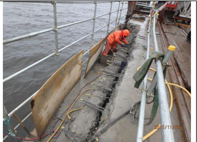
Removal of existing pier edge
