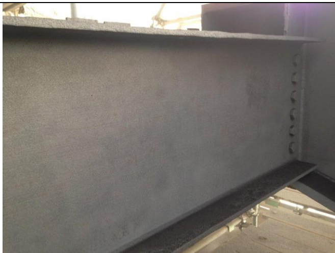
Steelwork following grit blasting
