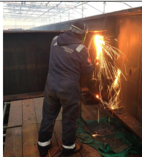
Linkspan steelwork repairs
