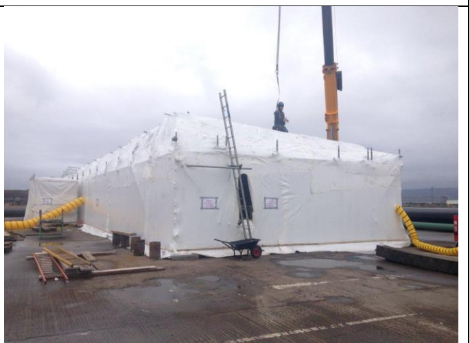
Completion of encapsulation of linkspan at Inchgreen
