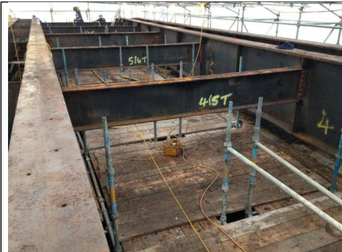
Linkspan structure within encapsulation- prior to grit blasting
