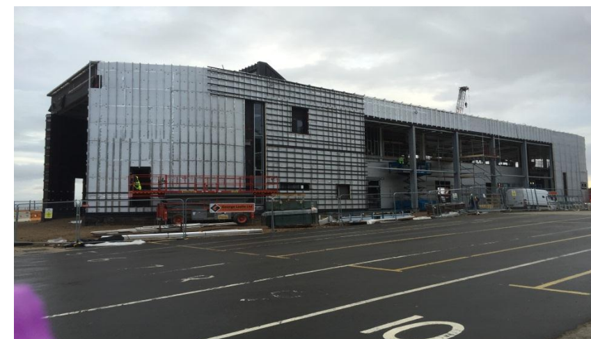
26/9/2016 Insulation and Framing South Elevation New Terminal Building
